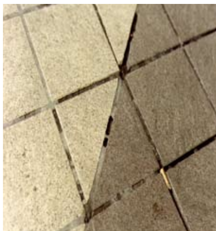
Pictured above: Tiles and grout cracking.
