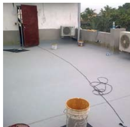
Pictured above: 300m² Butynol roof installation in Chennai.
