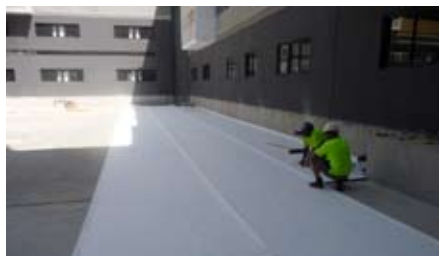
Pictured above: Membrane installation.
