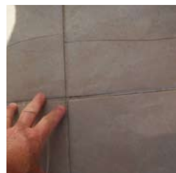
Pictured above: Cracking in the grout.
