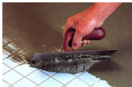
Pictured above: Applying Feather Finish over tiles for a smooth, even finish.
