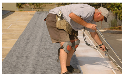
Pictured above: Unique ECO Butynol spraying system.
