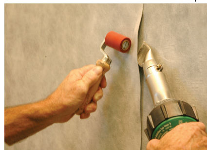
Pictured above: Undertile Butynol laps & seams are heat welded.
