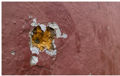
Pictured above: Foam penetrated by water, resulting in rot.
