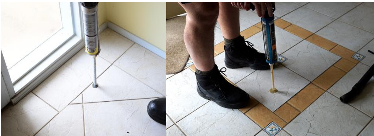
Injecting ARDEX RA56 at left and Dunlop Ardit Crack Filler at right
