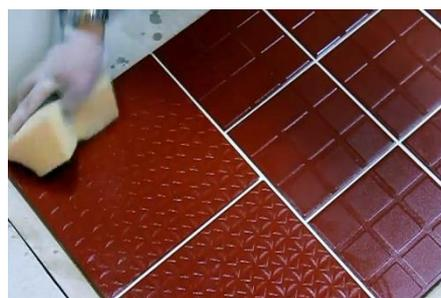
**TIP:** *A clogged sponge, ‘magic cloth’ or scouring pad will result in it dragging partially reacted epoxy grout out of the joints and depositing residue on the surface of the tiles. Use a small amount of household detergent or white vinegar (20ml in 5 litres) in clean water to wash the sponge and scouring pad to prevent epoxy residue build-up.*
